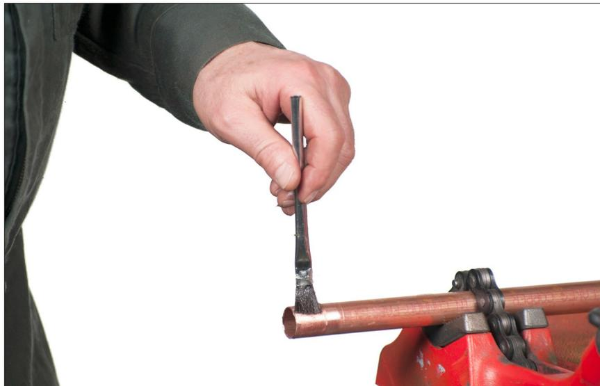
**Figure 6**—Flux will allow the solder to freely flow around the pipe.
