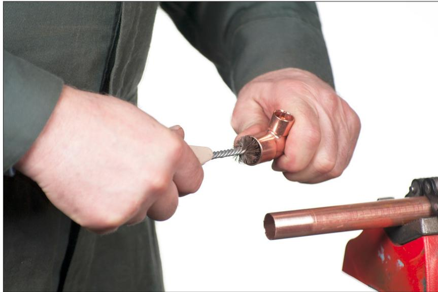
**Figure 5**—Polishing the inside of a fitting with a fitting brush. An alternate solution is to use sand cloth and a pinky finger.
