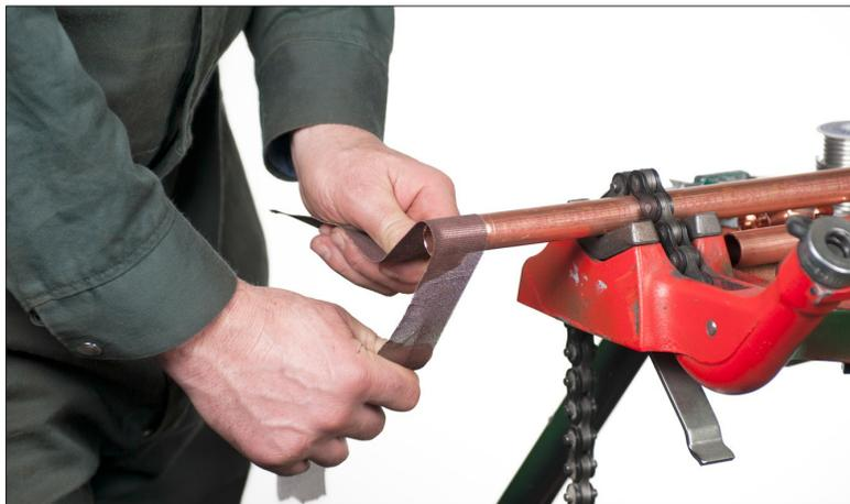
**Figure 4**—Polishing the outside of the pipe ensures good bonding between the pipe and solder.
