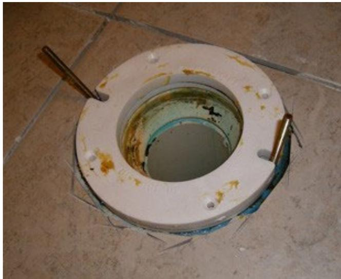
**Figure 8**—Brass closet bolts are aligned with the floor flange to secure the bowl to the flange.
