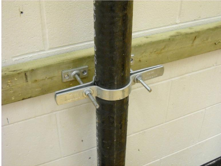
**Figure 16**—Vertical piping can also be supported by a riser clamp.
