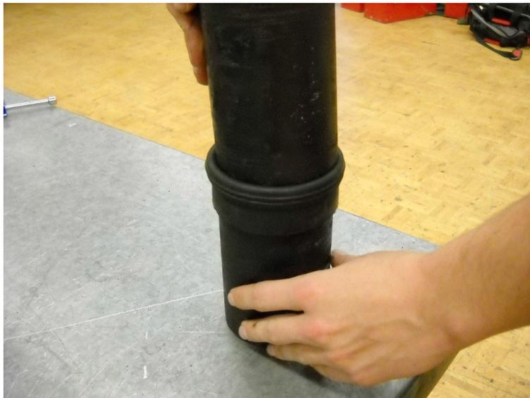
**Figure 4**—The top pipe should be fully inserted, then aligned straight.
