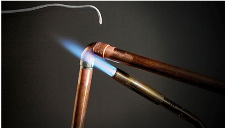
**Figure 7**—Heat should be applied at the centre of the fitting to draw the solder into the shoulder.
