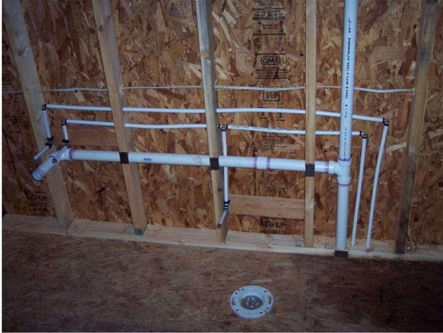
**Figure 24**—Drainage and water lines
