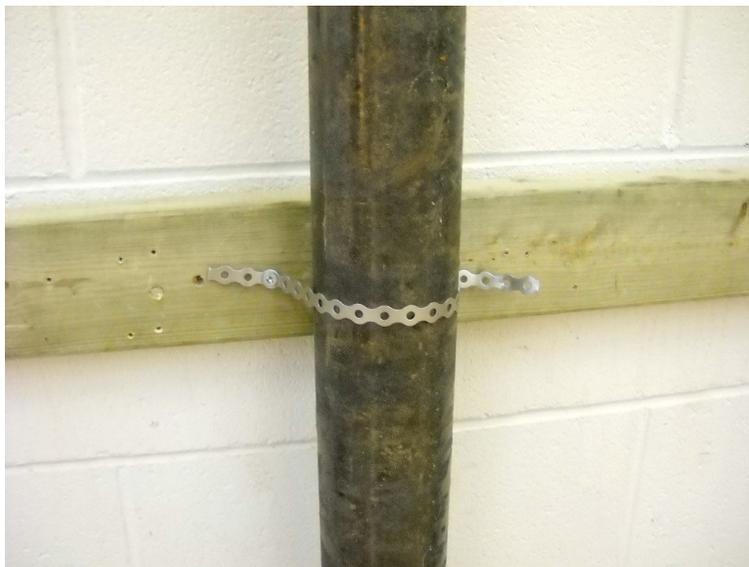
**Figure 15**—Strap iron is used in industry to support vertical piping.
