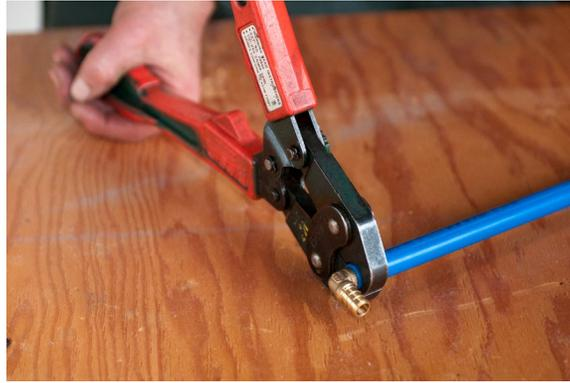
**Figure 14**—Using the crimping tool
