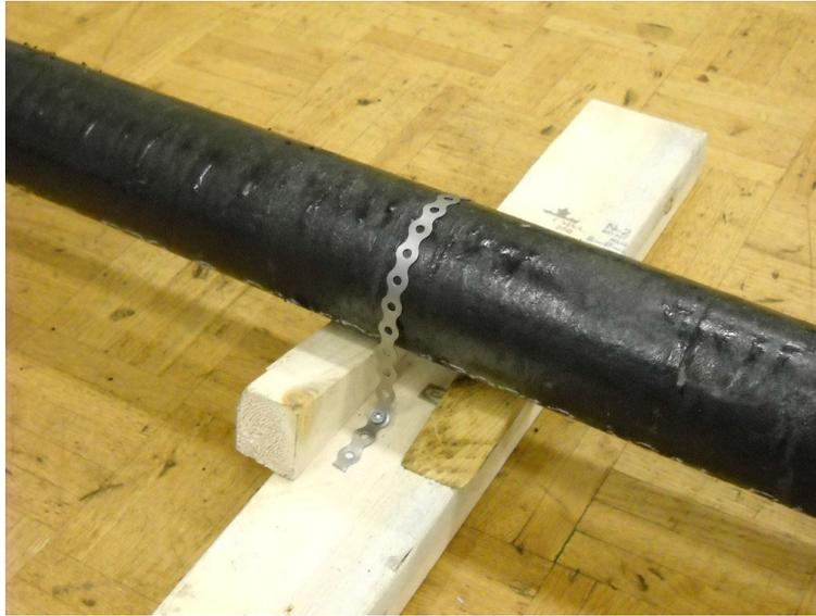
**Figure 14**—Wooden wedges and strap iron grade this cast iron in a shop environment.
