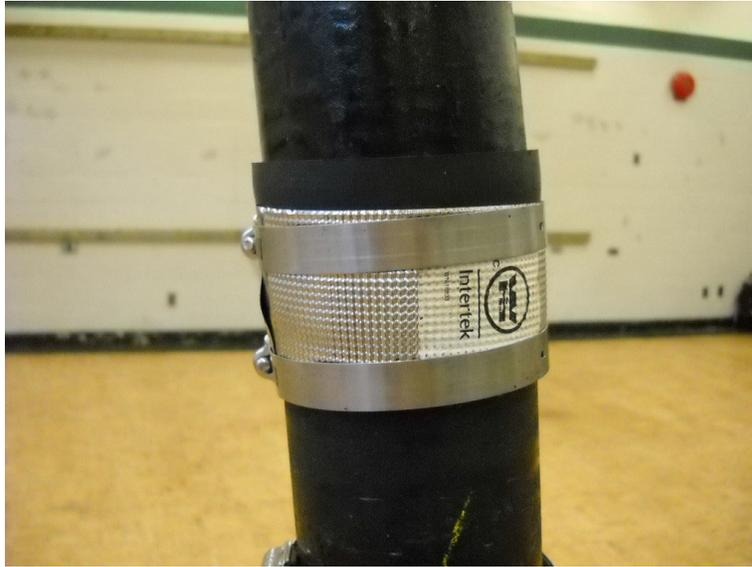
**Figure 6**—An example of a poorly installed clamp. The stainless steel band will not generate enough pressure to create a watertight seal.
