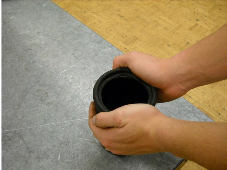
**Figure 3**—Rolling the rubber gasket allows a pipe or fitting to be easily inserted into the gasket.
