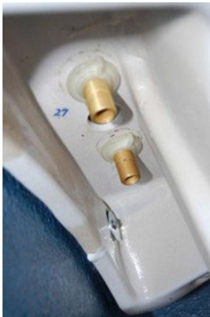
**Figure 9**—Faucets are normally connected to the basin by means of a threaded nut. Braided water supply lines run from the brass connections to the CR 19 stops.
