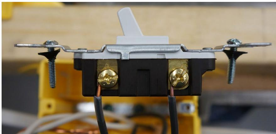
**Figure 23**—Proper installation under terminal screw
