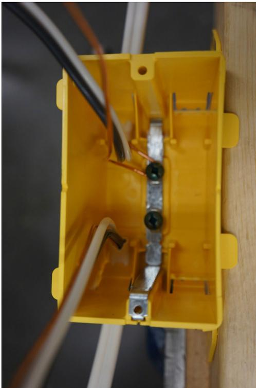
**Figure 13**—Box showing the ground wire looping around the grounding screw
