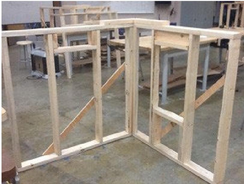
**Figure 1**—Sample wall section
