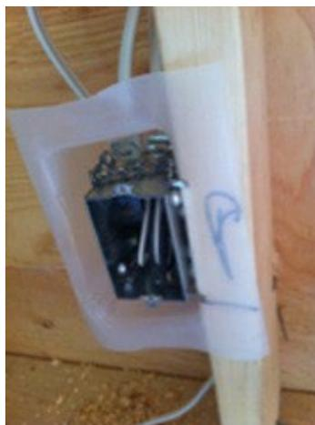
**Figure 4**—Vapour barrier example
