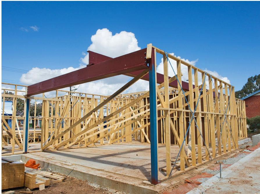
**Figure 6**—Typical temporary bracing of a wall section after checking for square and for plumb
