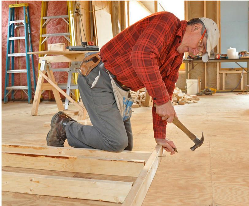
**Figure 4**—Typical nailing procedure for a wall
