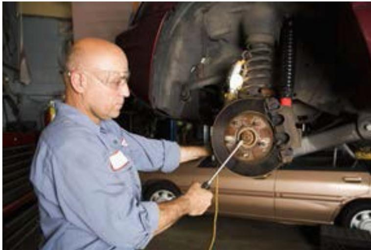
**Figure 1**—Wearing eye protection for a brake job
