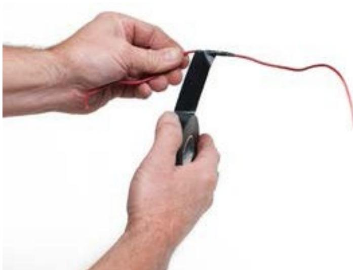
**Figure 6**—Finish by ending on the wire insulation on the other side.
