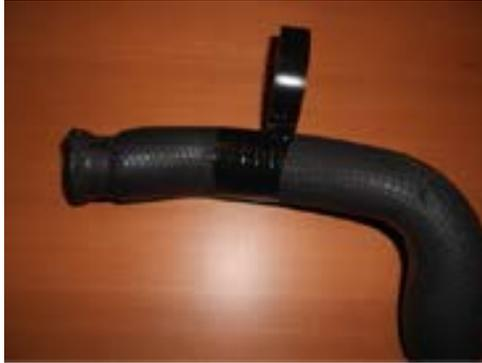
**Figure 10**—Wrapping electrical tape
