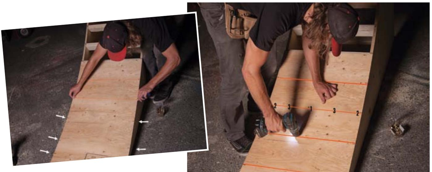
**9.** Add screws in all ribs, first in the centre, then one on either outside edge, then add screws in between each of the previous screws. This will help prevent warping.
