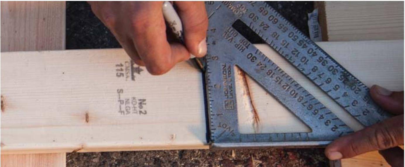
4. Before you cut your ribs, double check your rib measurements. If they are correct, place 2 of your scrap 2x4s underneath to lift the wood you will be cutting off of the ground. Make sure your supporting 2x4 or work surface is not going to interfere with the saw when it passes over your cut line.
